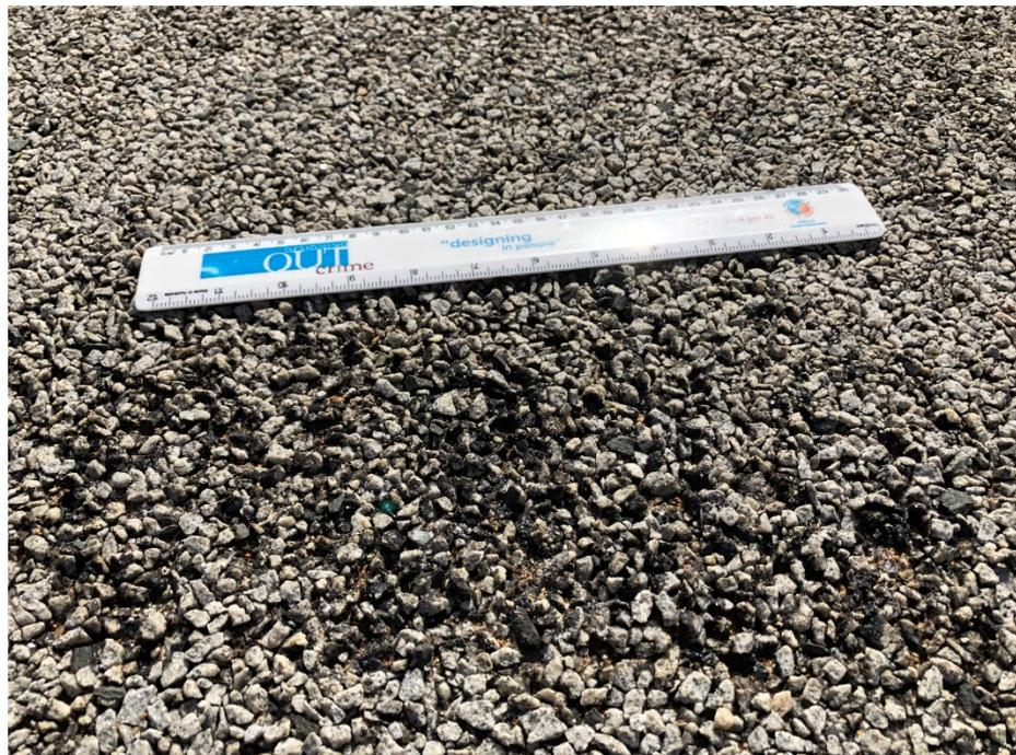
Enquiries regarding these scuff marks conclude that this is likely the source of the loose stone and is caused by turning plane wheels under normal operating conditions.
