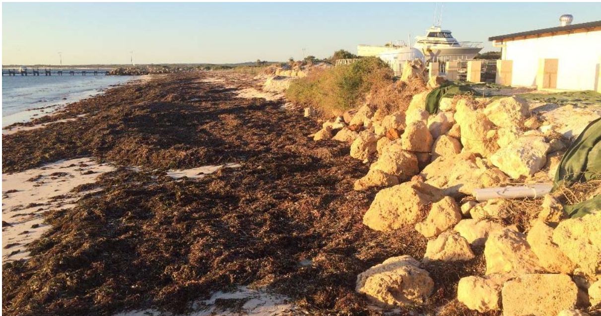
Figure 5-1 Small section of seawall in front of Indian Ocean Rock Lobster property
