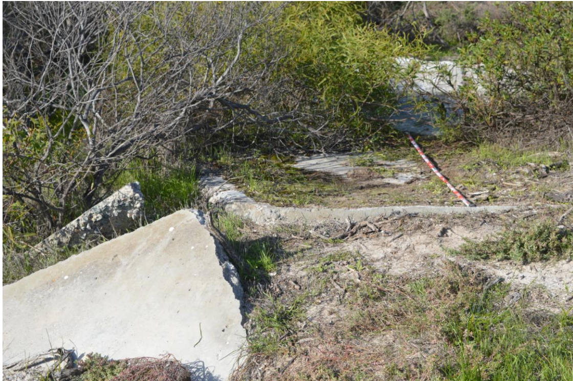
Figure 15: Foundation Two concrete foundations. Scale 2m. Photo facing north.
