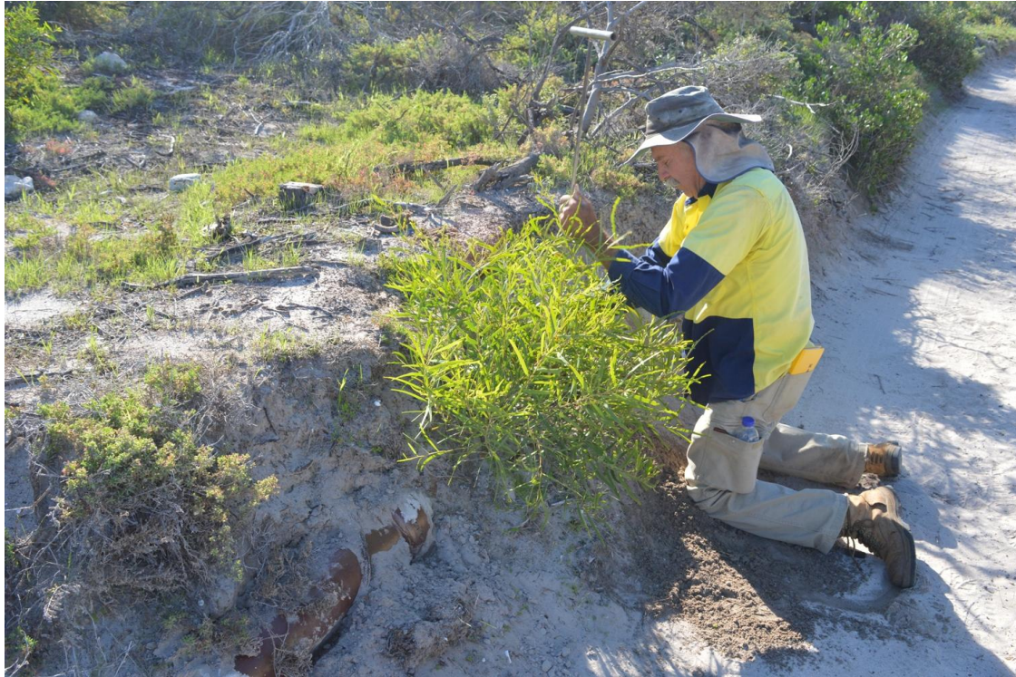
Figure 24: Geoff Royce inspecting the section of earthenware pipe that is visible from the vehicle track. Photo facing northwest.
