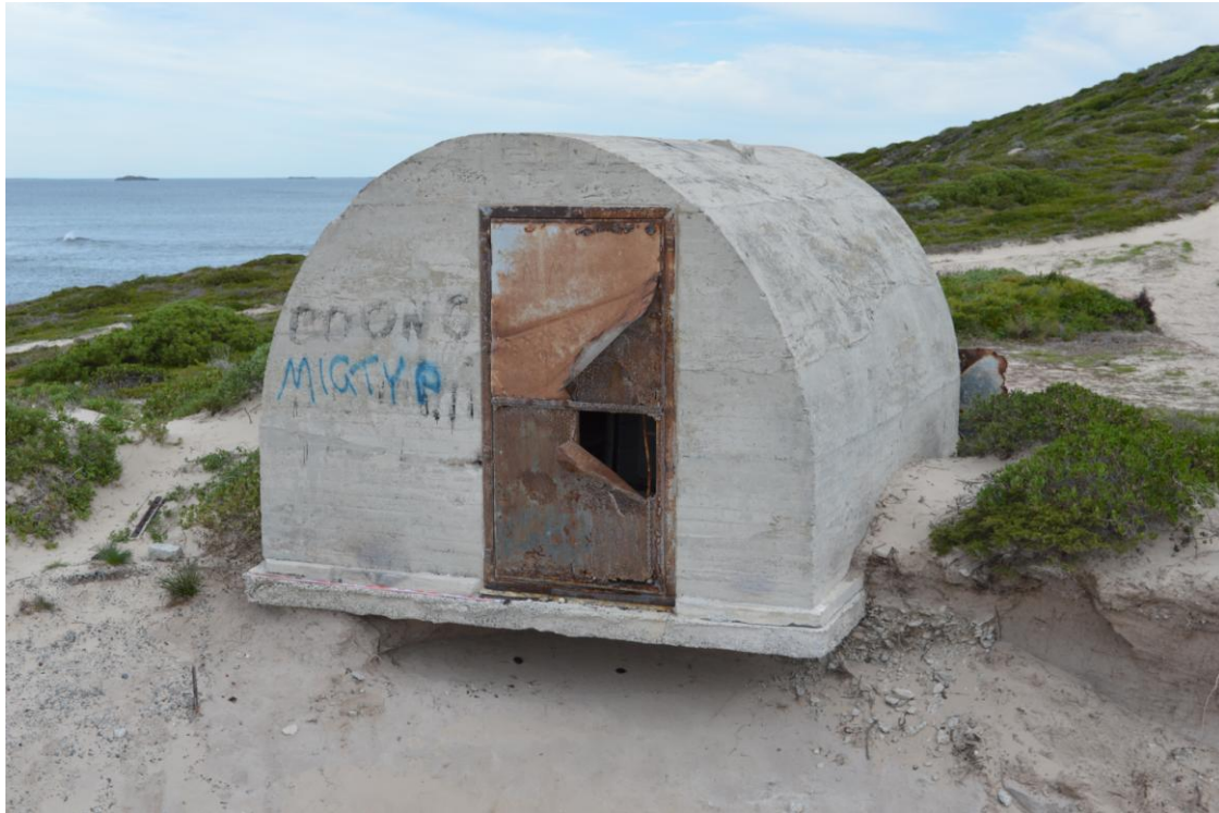
Figure 6: Igloo A. Photo facing south.
