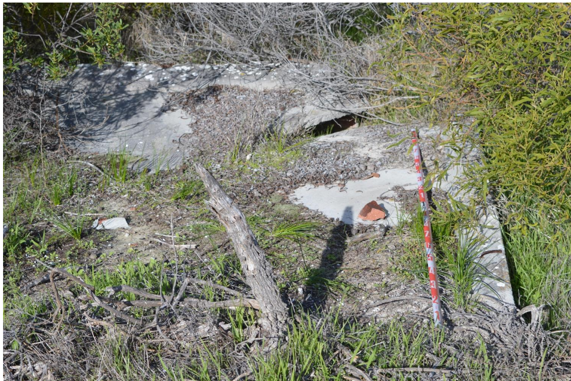
Figure 14: Foundation Two concrete foundations. Scale 2m. Photo facing east.
