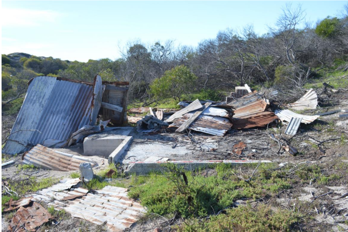
Figure 16: Foundation 3 concrete foundations overlain by rusted iron corrugated sheets. Scale 2m. Photo facing north.
