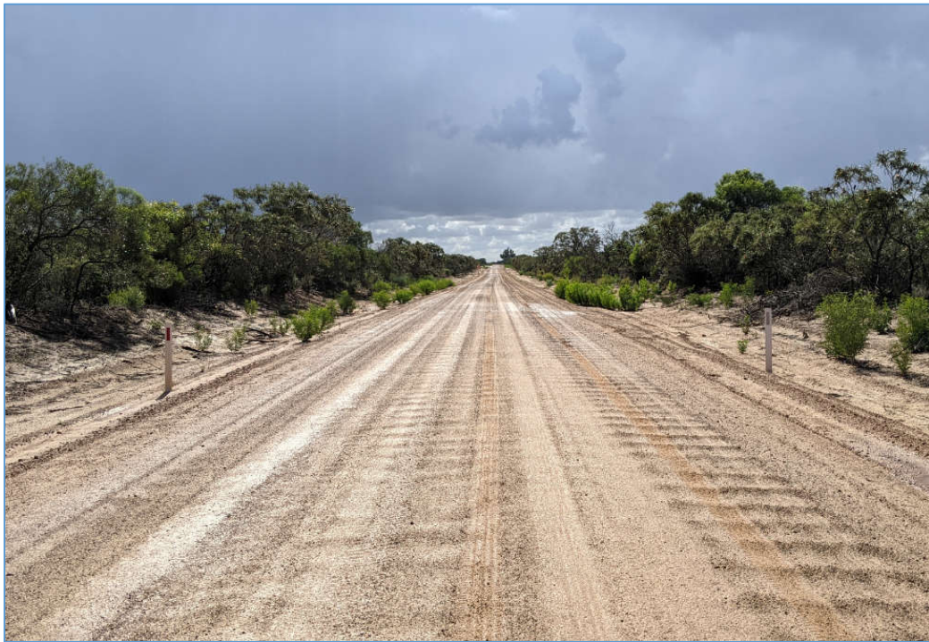
Figure 31: Typical Existing Munbinea Road Unsealed Formation – Example 1 (SLK 0.21)
