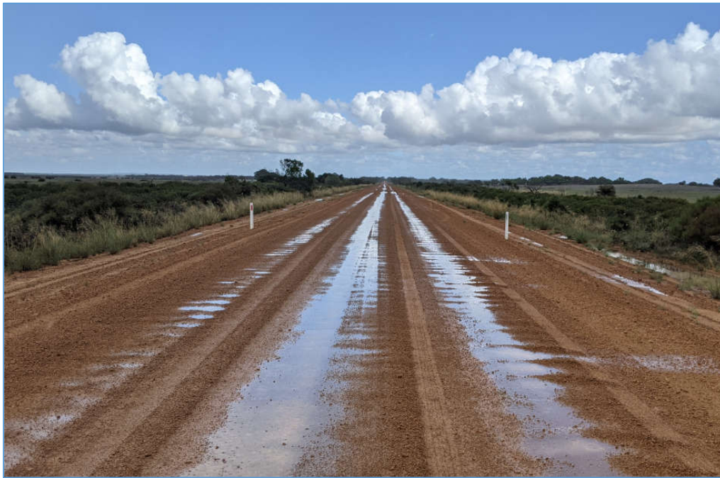
Figure 33: Typical Existing Munbinea Road Unsealed Formation – Example 3 (SLK 9.90)
