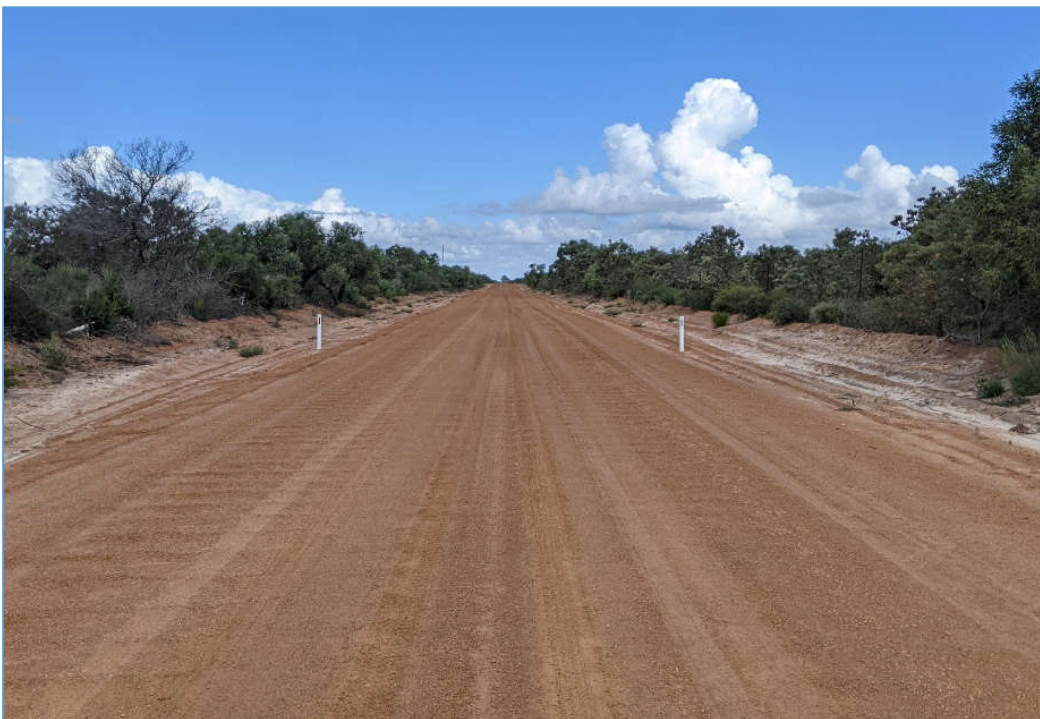
Figure 32: Typical Existing Munbinea Road Unsealed Formation – Example 2 (SLK 2.55)
