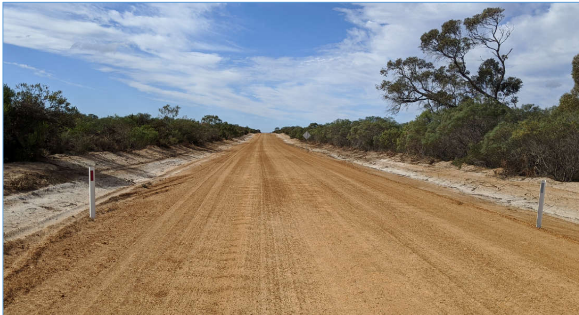
Figure 25: Typical Existing Wongonderrah Road Formation
