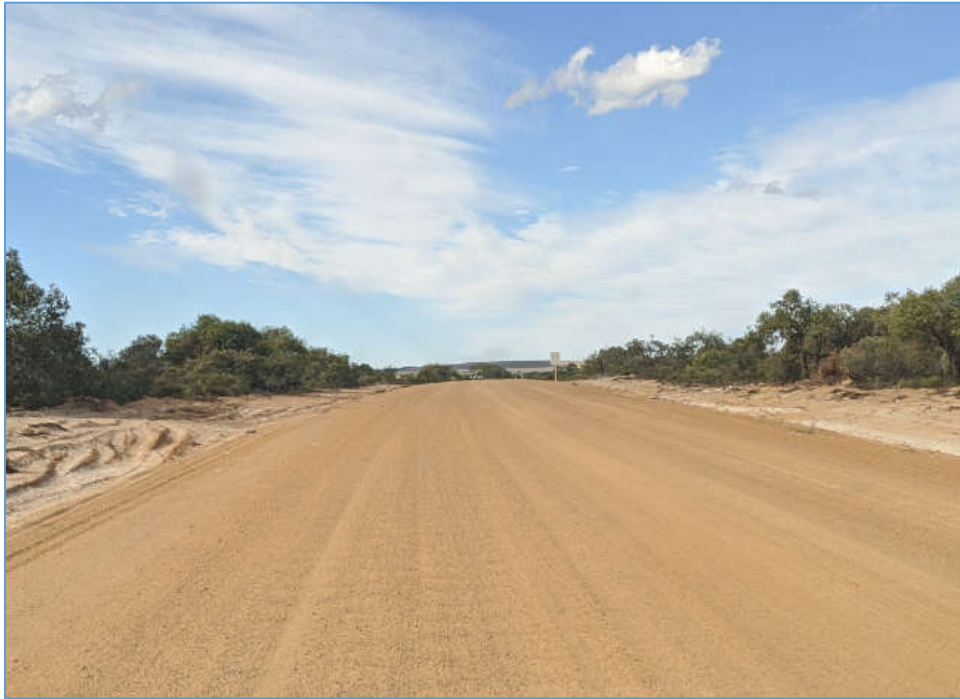
Figure 20: Approach Sight Line to Brand Highway – Prior to Crest
