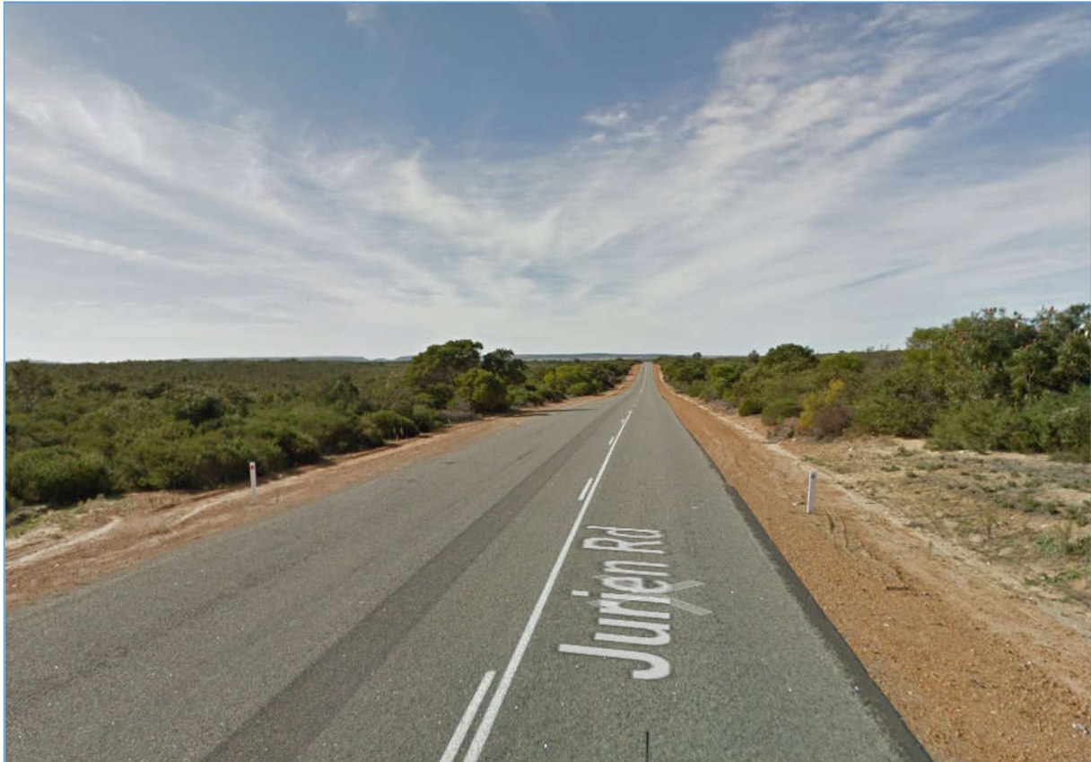
Figure 46: Typical Existing Jurien Road Formation
