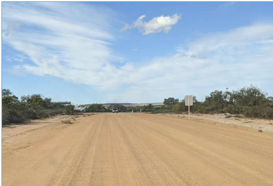
Figure 21: Approach Sight Line to Brand Highway– After Crest
