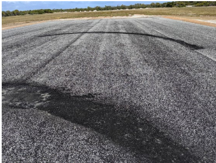
Turing C130 surface damage
