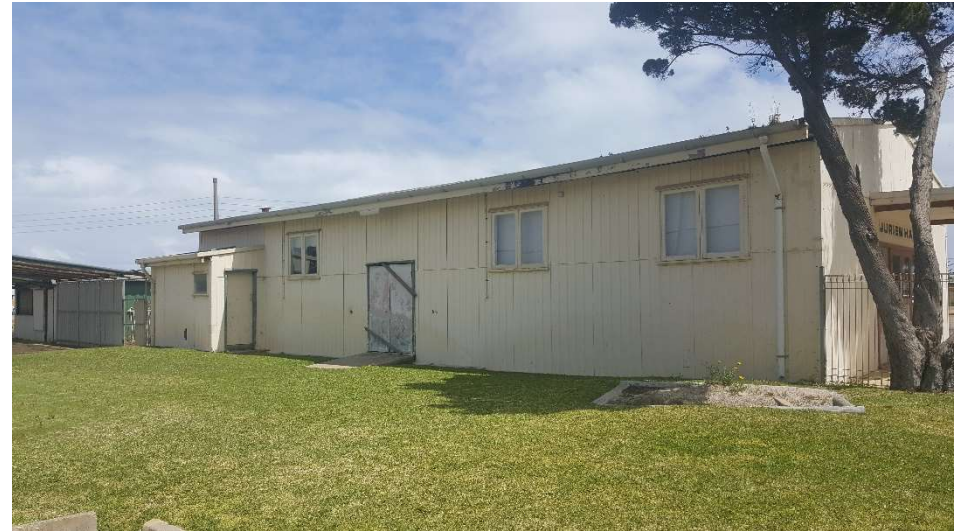
Photograph 4 – Overall view of the hall looking toward the South
