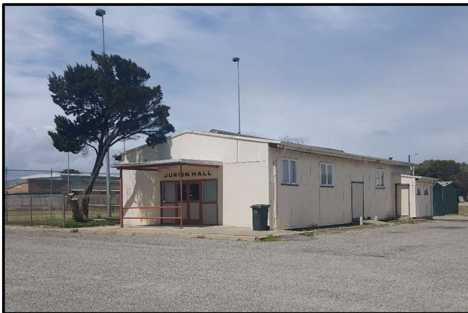
Figure 1 : Photograph of the town hall taken during WML Consultants inspection.
