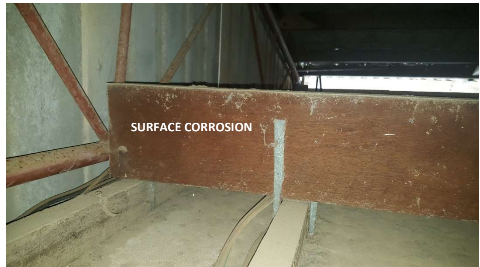
Photograph 24 – Within the roof space view on the gable facing the Southeast
