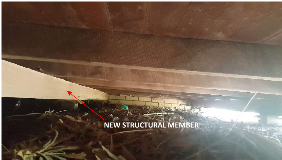
Photograph 9 – View to the underside of the Hall floor looking East
