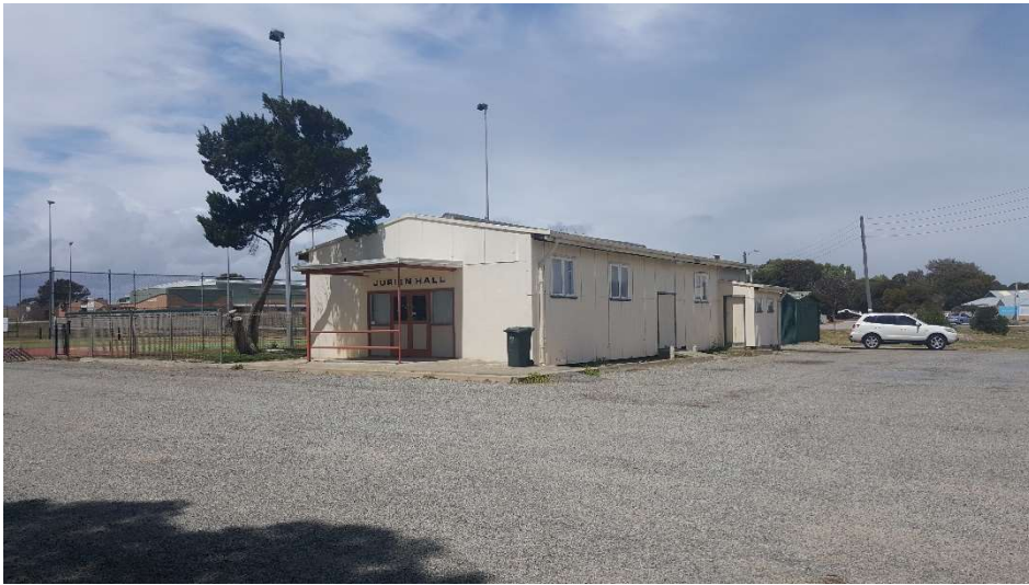
Photograph 1 – Overall view of the hall looking toward the Northeast
