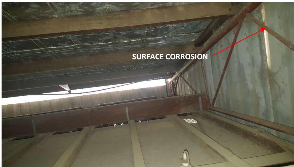
Photograph 23 – Within the roof space view on the gable facing the Northeast
