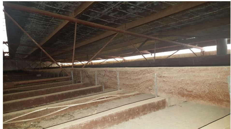
Photograph 22 – Within the roof space viewing toward the Northwest.
