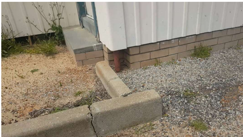
Photograph 7 – Column support for upper roof at toilet external entrance.
