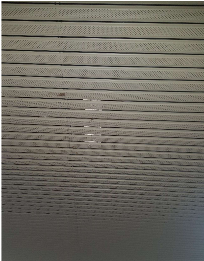
Photograph 19 – Perforated ceiling cladding viewing to the roof structure
