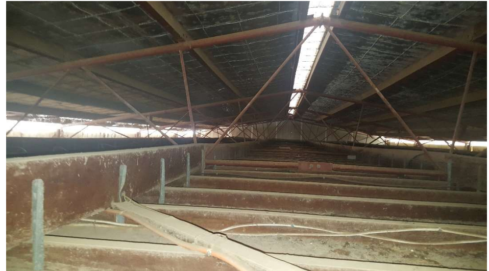
Photograph 20 – Within the roof space viewing toward the West.
