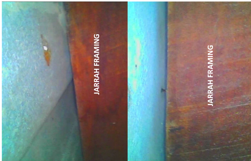
Photograph 17 – Bore Scope placed within the wall (Penetrated sections of wall sheeting).
