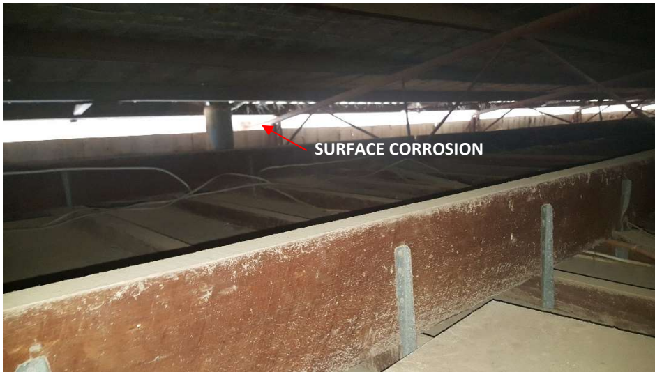
Photograph 21 - Within the roof space viewing toward the Southwest.
