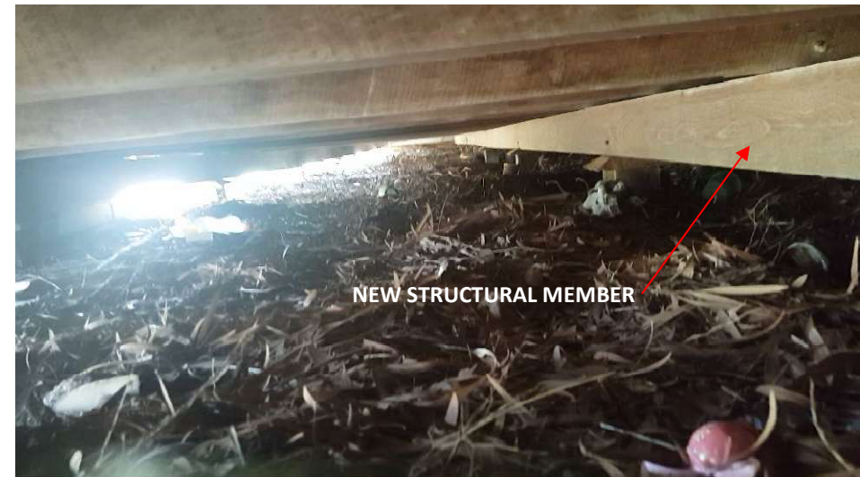
Photograph 10 – View to the underside of the Hall floor looking West
