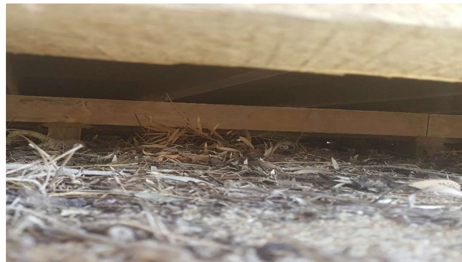
Photograph 8 – Floor joists supported on secondary Jarrah beams seated on stub supports
