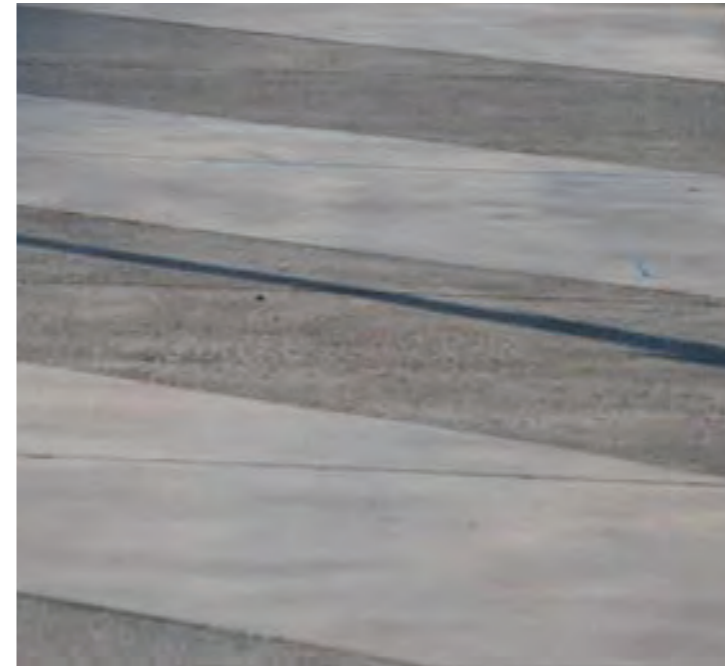
Trafficable Sand Blasted
