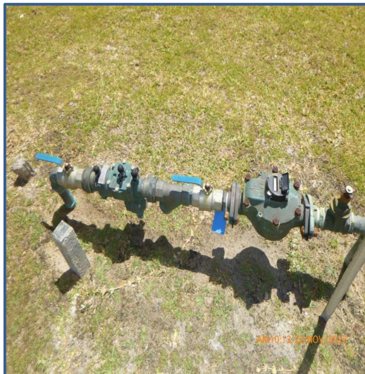
L 2: Reduced pressure zone device (RPZD) temporary node logging residual pressure ONLY during testing
