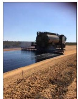
Works entailed ripping, reconditioning and widening of the existing pavement to 10m width. Importation of gravel to build the road pavement up to required levels. Extensions to existing culverts and improvements of roadside drainage. Water binding and compaction of pavement ready for seal. Primer seal of 10mm aggregate this year, to be followed by a final coat seal of 14mm aggregate next year with new line marking.
