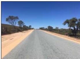
Reconstruction of Jurien East Road commenced in January 2017. This entailed widening of the road from a seal width of 6m or less in places out to 8m. The first stage of this project entailed commencing at the Brand Highway and working back for 7km. It is proposed to progressively continue widening of this road in various stages heading in a westerly direction, with proposed intersection improvements at Black Arrow Road as well as the Munbinea and Cockleshell Gully Road intersections.
