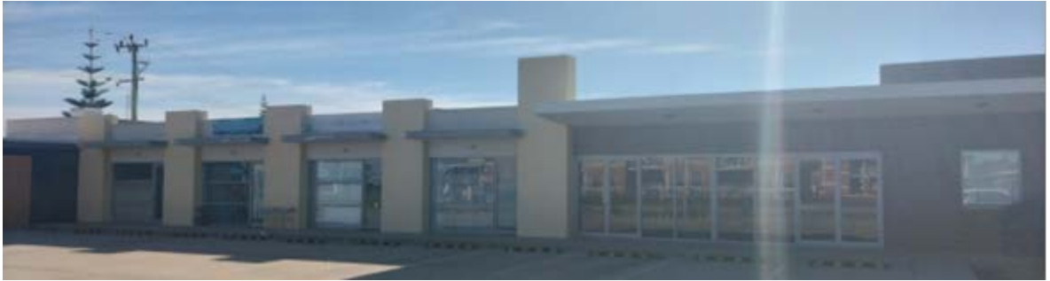
Jurien Central Murray Street Frontage
