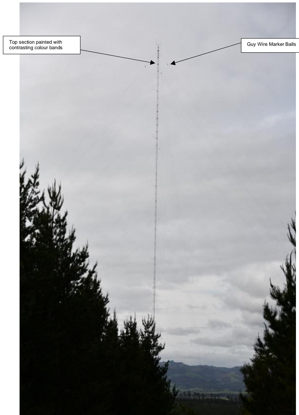
Figure 8 – An appropriately marked Meteorological Monitoring Mast 22
