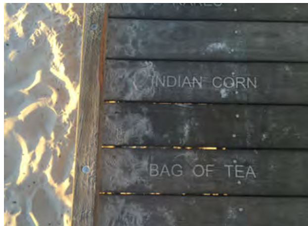
Image 37. Etching to timber deck Source: UDLA
