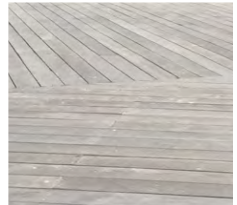
Timber deck and boardwalk
