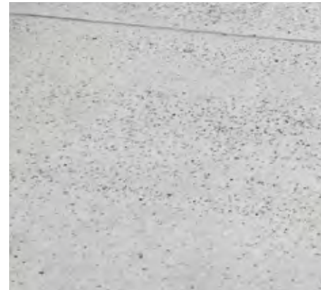
Salt seeded concrete
