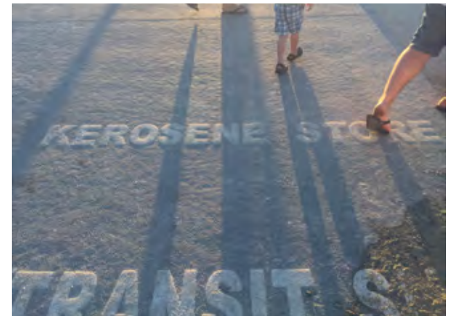
Image 36. Sandblasting in concrete paving Source: UDLA
