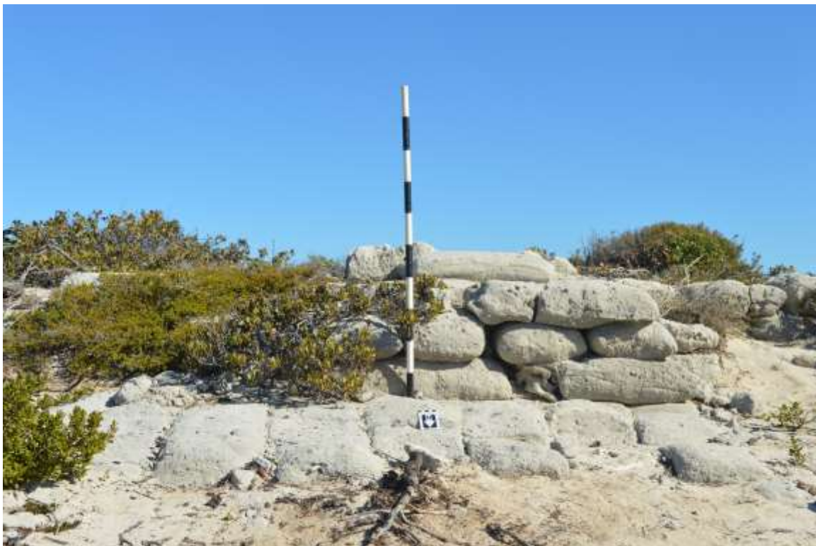
Figure 6. Sand bag steps at 'Doover' site showing heights (100mm increments). HDA photo.
