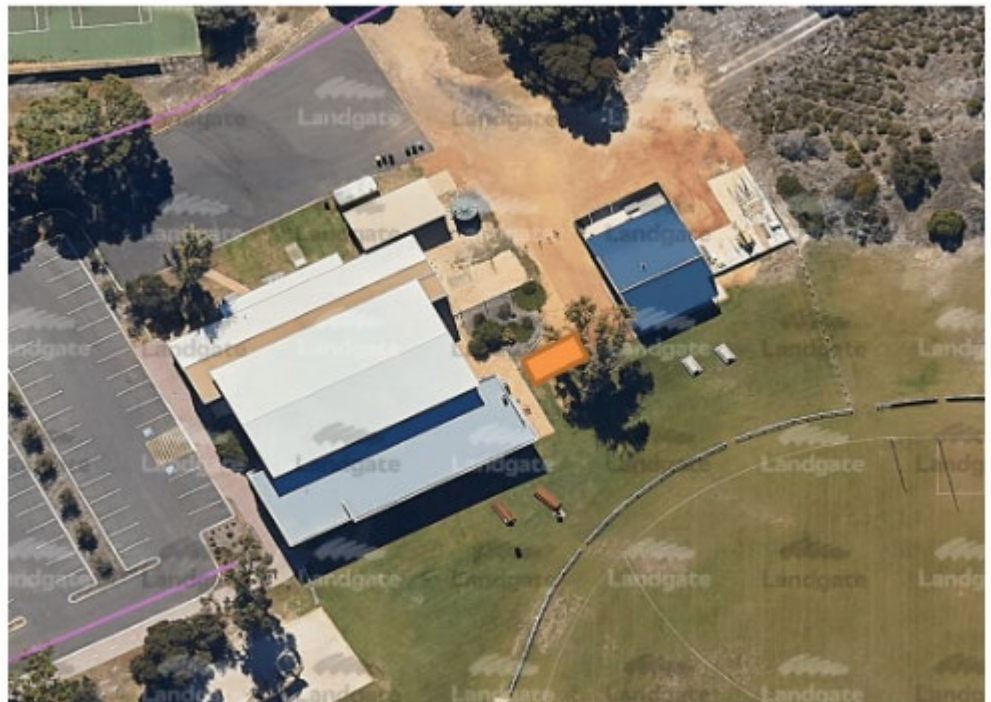
Cervantes Recreation Centre & Cervantes Football Club Changeroom with the proposed development shown by the orange rectangle.
