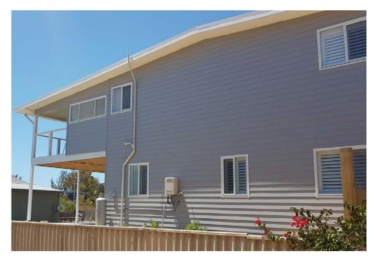
The ground floor windows have been obscured glazed and timber screened internally after consultation with the owner builder. While the first floor windows are above 1.6m in height and do not require screening although internal timber screens have been provided to one of these windows as seen.
