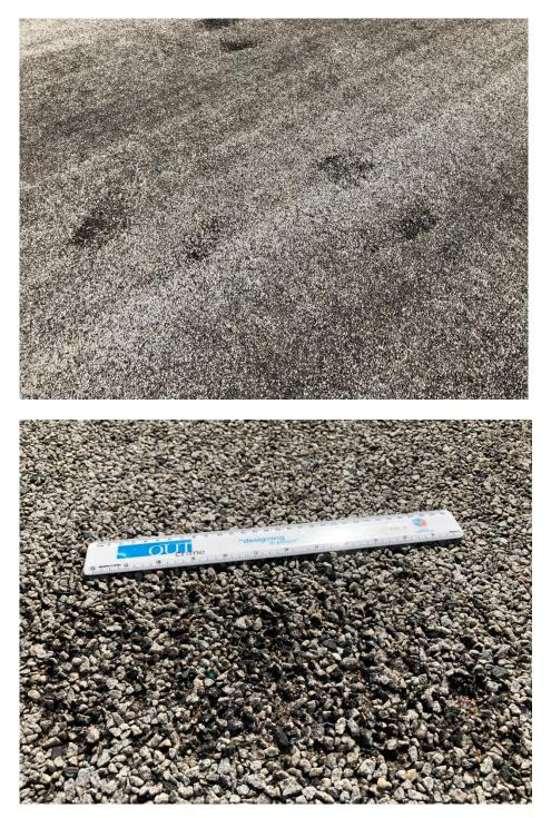
Enquiries regarding these scuff marks conclude that this is likely the source of the loose stone and is caused by turning plane wheels under normal operating conditions.
