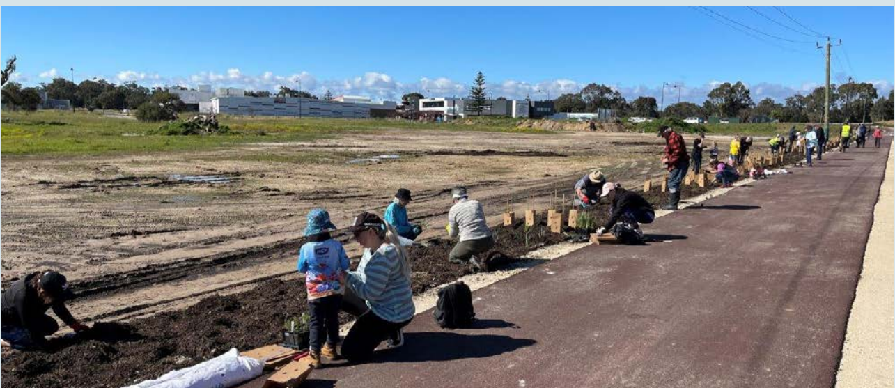
Buayanyup Drain Path. Credit: City of Busselton
