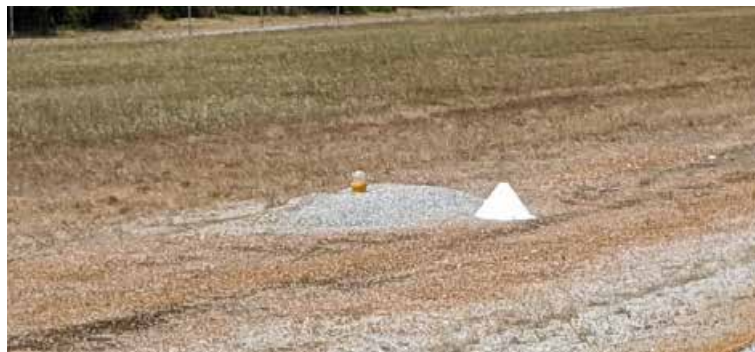
Light surrounded by aggregate pile
