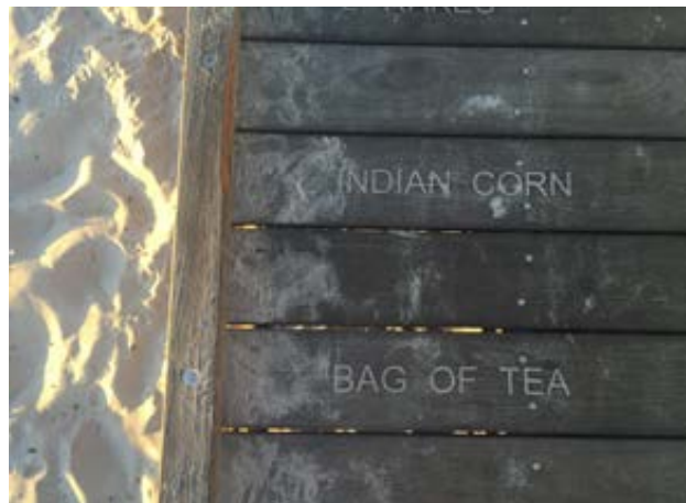
Image 37. Etching to timber deck Source: UDLA
