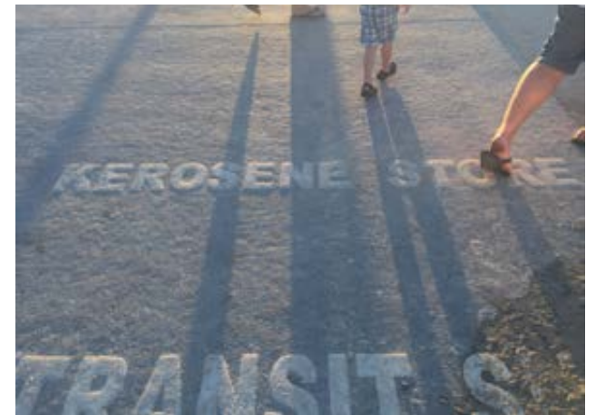
Image 36. Sandblasting in concrete paving Source: UDLA
