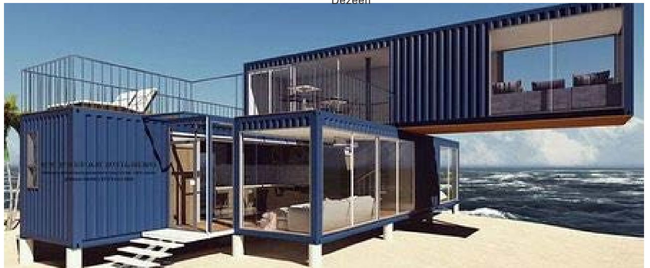
Image 19. Shipping container construction Source: Pinterest
