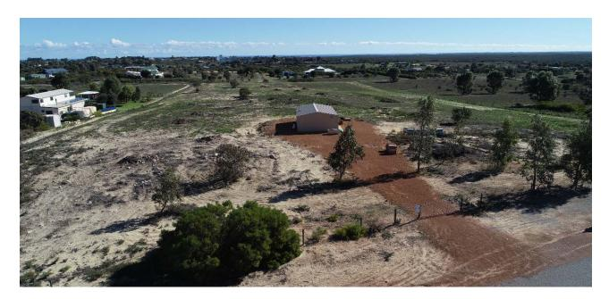
The existing shed has a wall height of 3m and a ridge of 3.8m. The proposed will increase this by 1.2m and 1.7m respectively. The area will also increase by 210m<sup>2</sup>, the majority of this being in front of the existing footprint.
