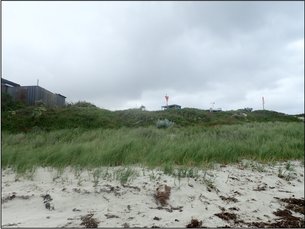
Figure 7 Typical perspective looking east from the Settlement beach illustrating the ability of the terrain, structures and vegetation to screen the guyed mast from view
