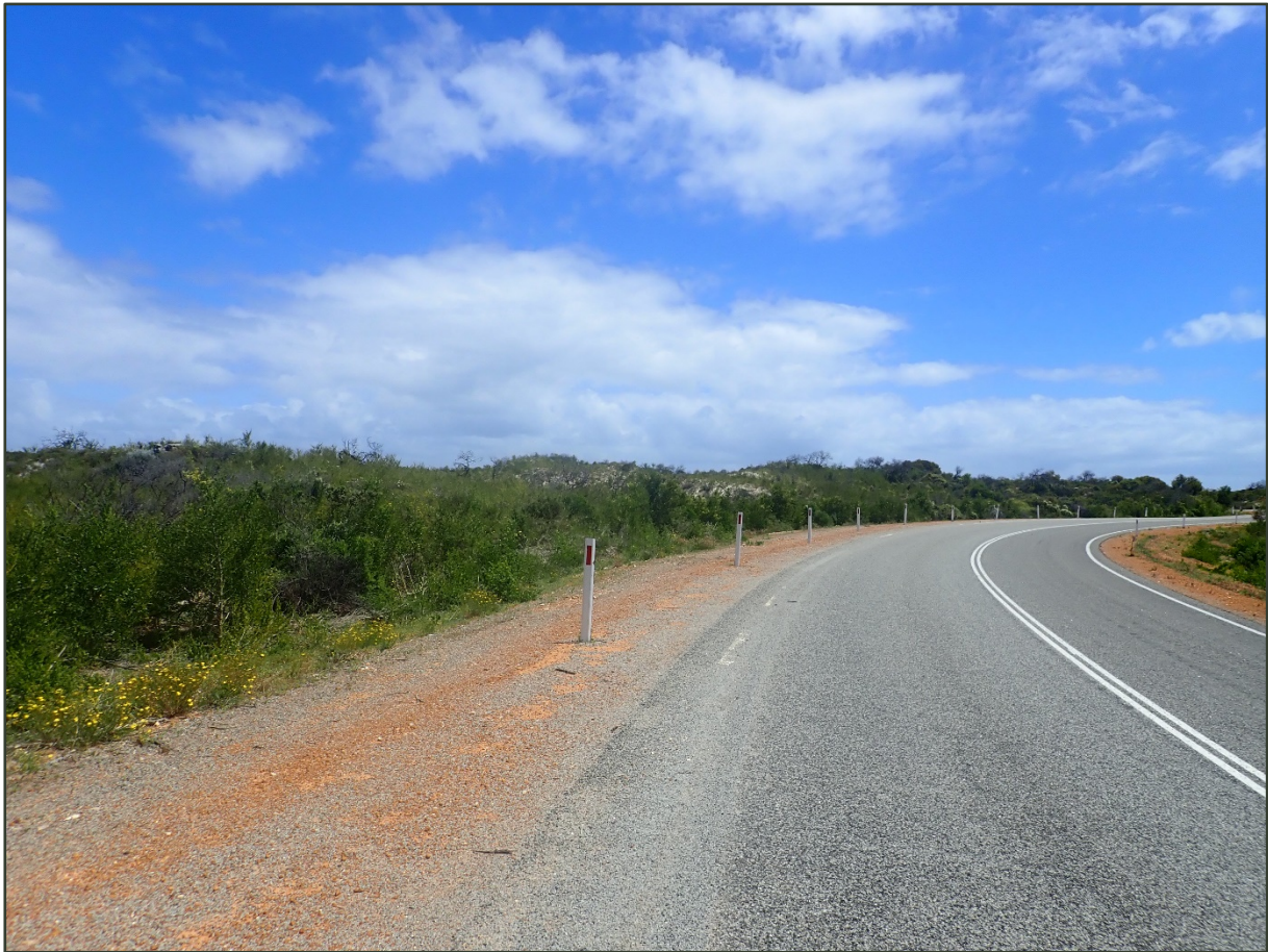
Figure 22 Photo location 19 Grey Settlement access road looking towards the proposed facility
