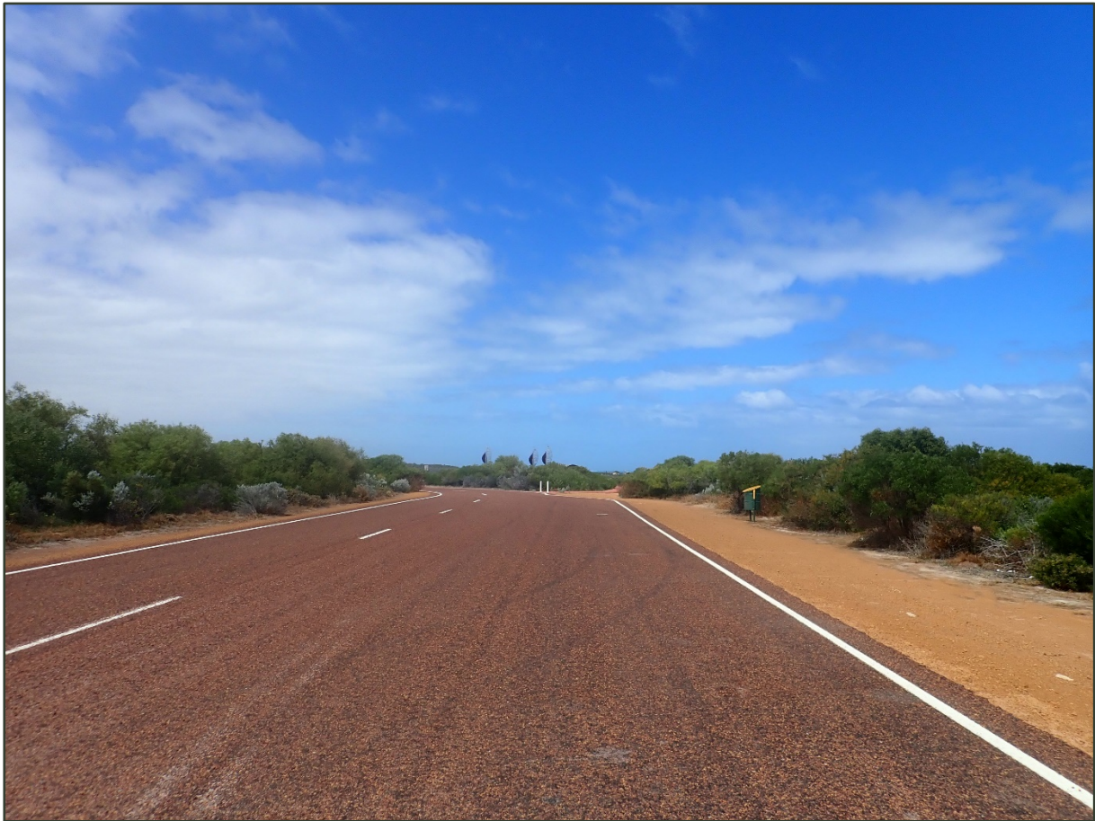
Figure 20 Photo location 13 looking southwards from the driver layover area
