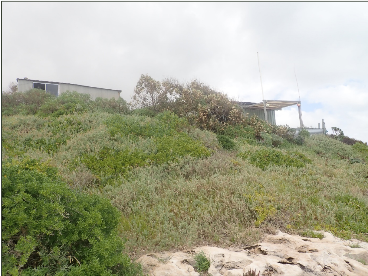
Figure 21 Photo perspective 59 looking towards the proposed facility from the beach
