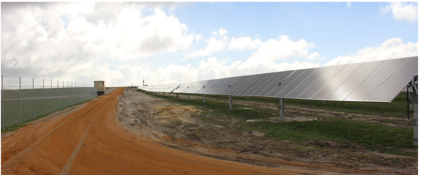
Emu Downs Solar Farm
