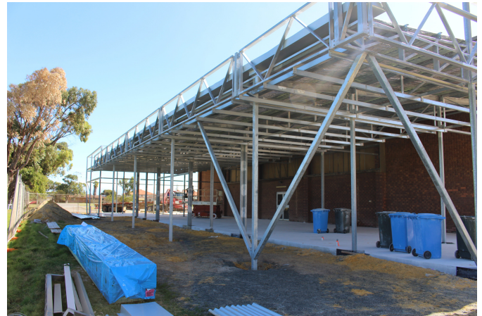
Construction of the Cervantes Multi Purpose Performing Arts and Cultural Centre
